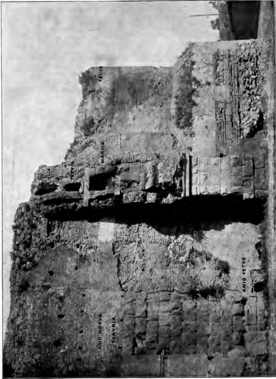
MARCIA, TEPULA OVER IT, AND JULIA OVER TEPULA ; and four other aqueducts, near Porta Maggiore.
